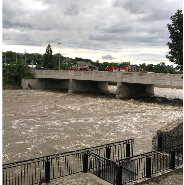
June, 2017 - Parkhill Road Bridge, Cambridge
